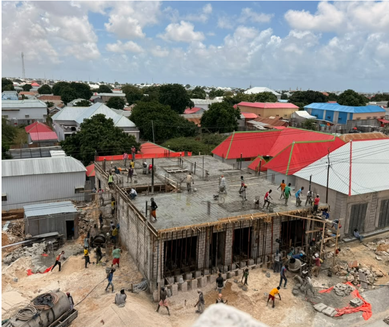
03 / CONCRETE STRUCTURE & FORMWORK
