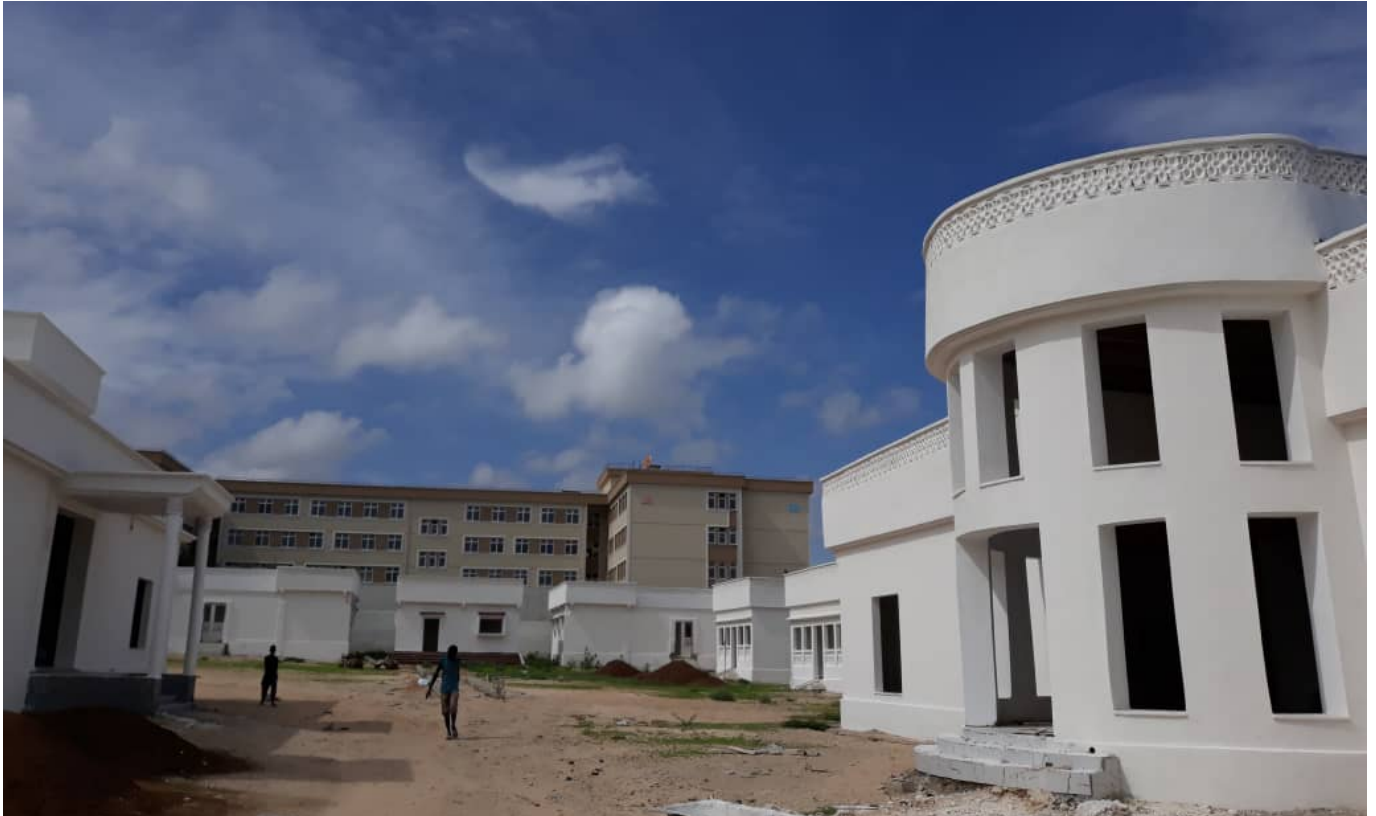
07 / COURTYARD & EXTERIOR WORKS
